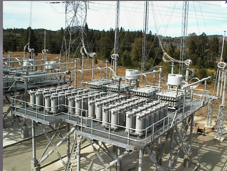
Typical series compensation (Courtesy of ABB)
