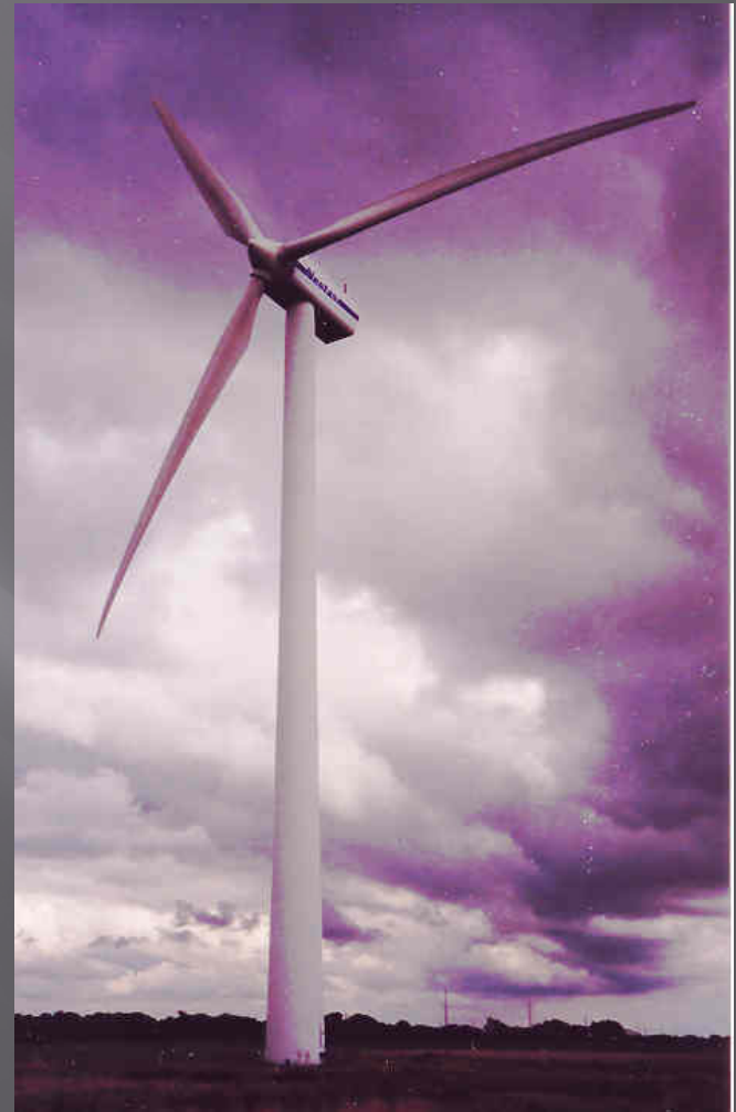
Vestas DFIG Wind Turbine Generator in Denmark
