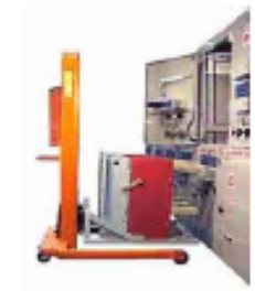
4. Lift Truck & Switchgear Position
