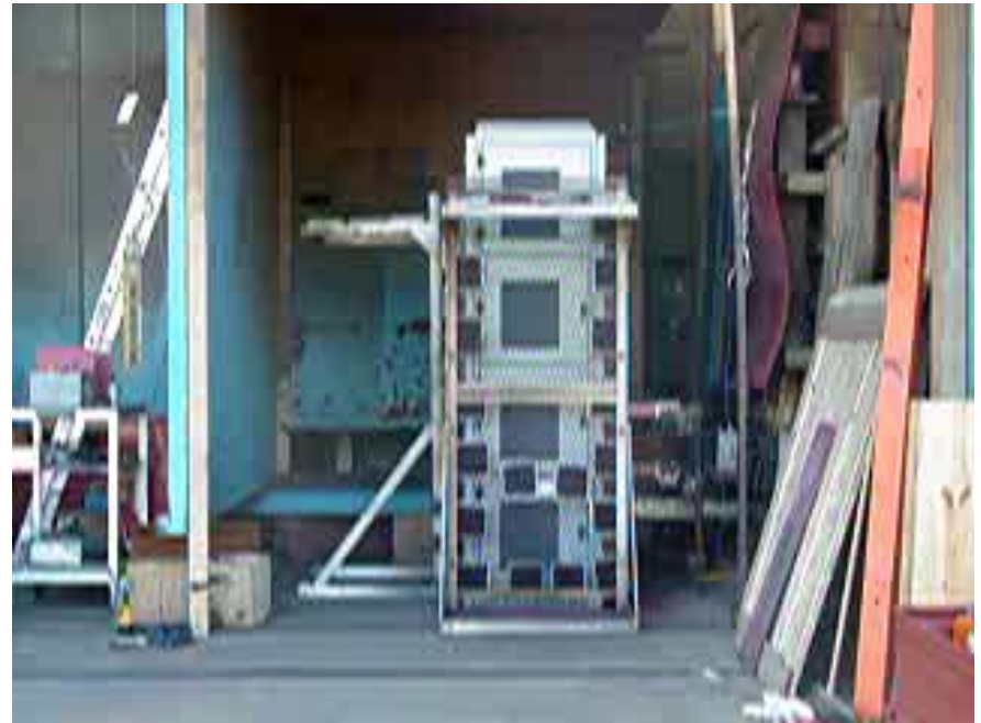
Insulated Main Bus 85kA 635V 13.7msec 13.2psi
