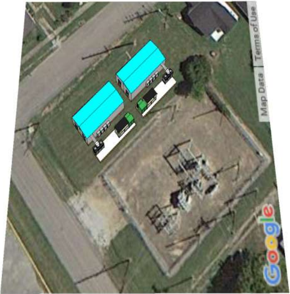
Courtesy of Siemens
