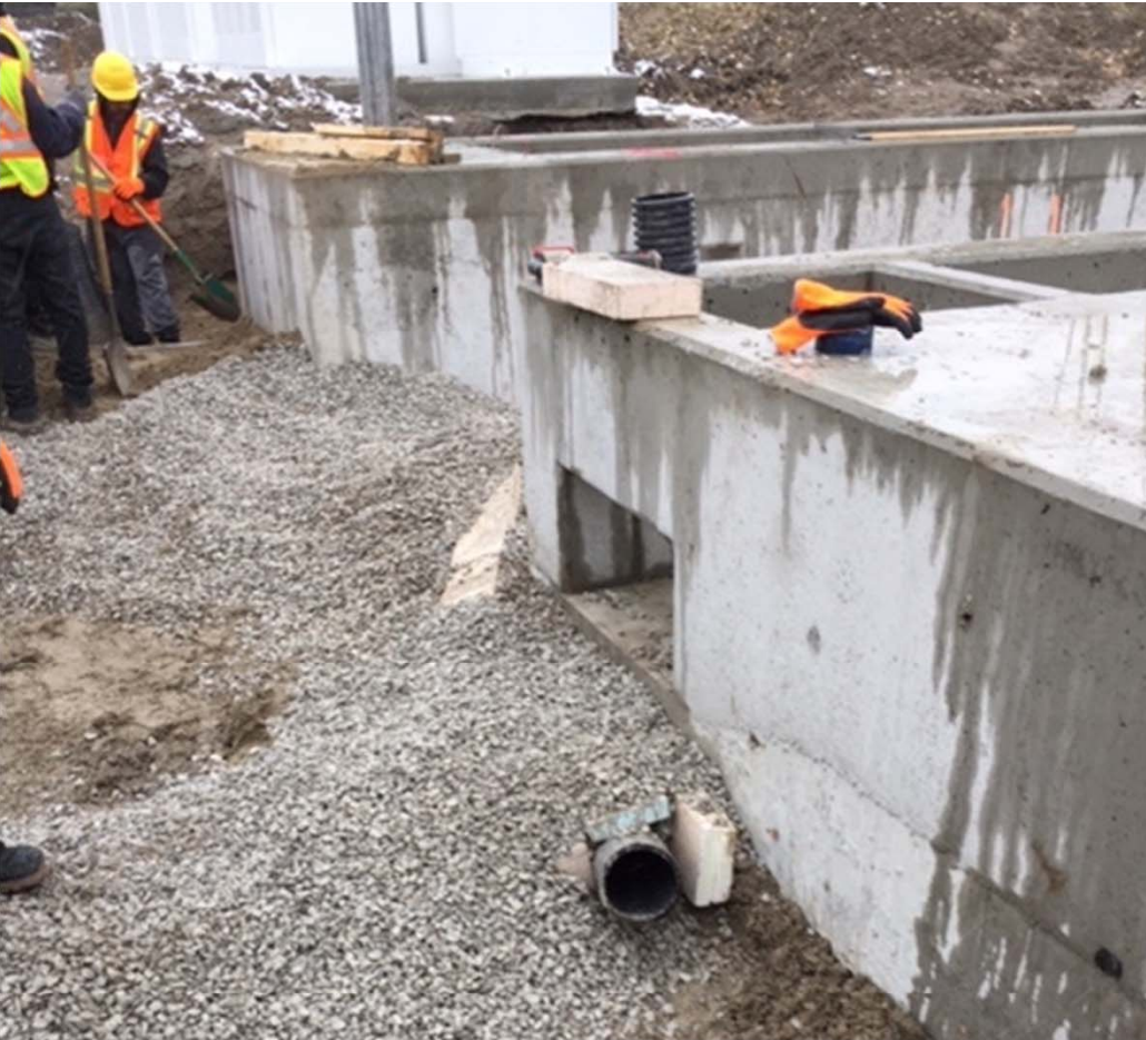
Installation: Trench Preparation
