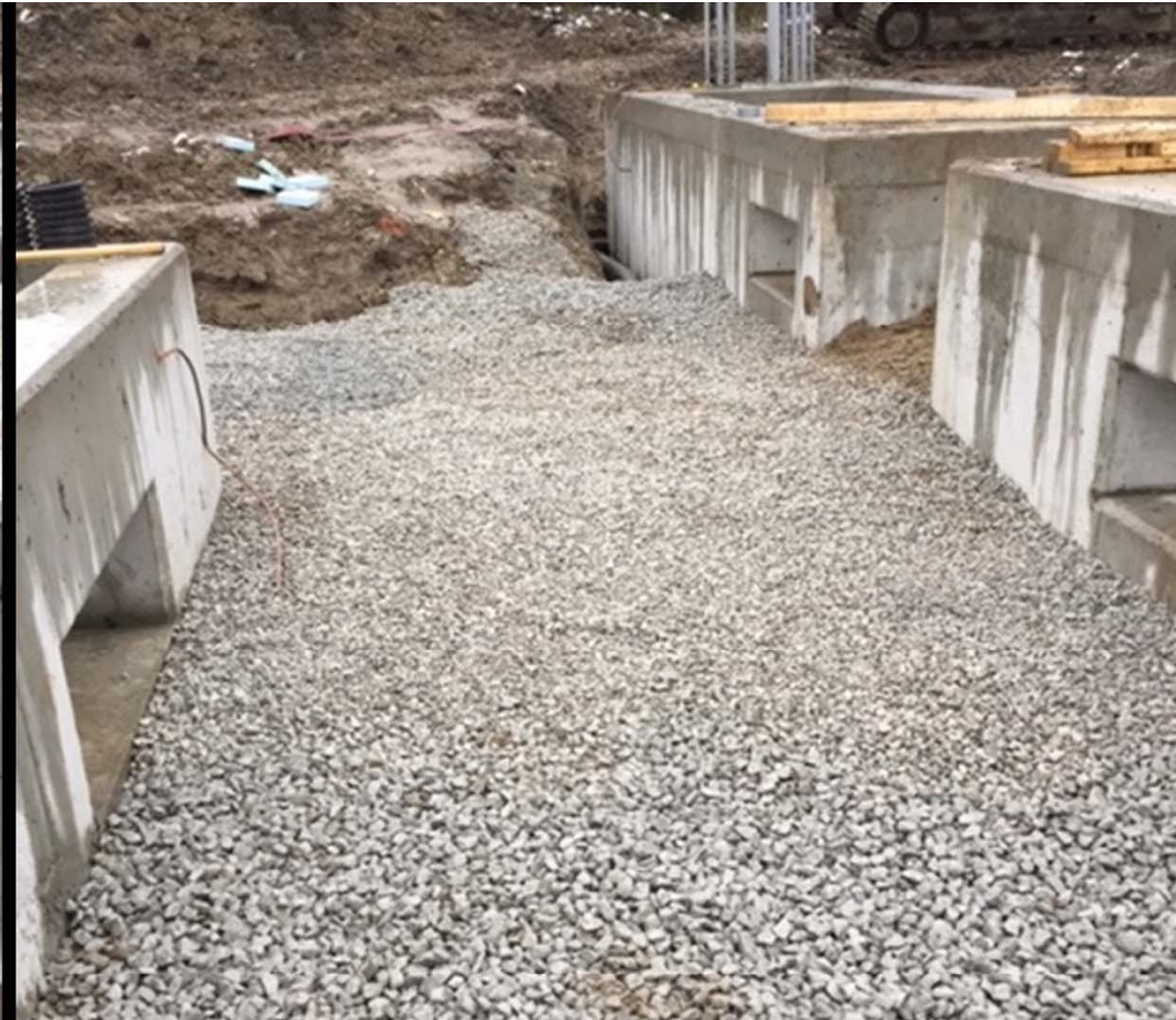
Installation: Trench Preparation
